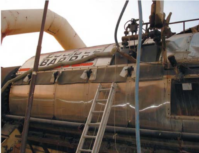
Fiber and sasobit are being fed into the mix.
