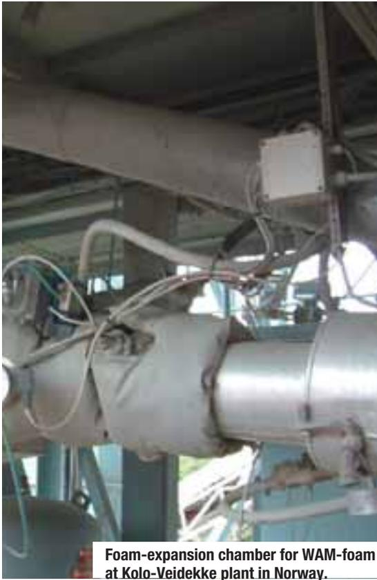
**Foam-expansion chamber for WAM-foam at Kolo-Veidekke plant in Norway.**
